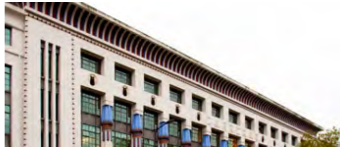
Existing building features a classic Art Deco cornice motif, as seen on former Carerras Cigarette factory
