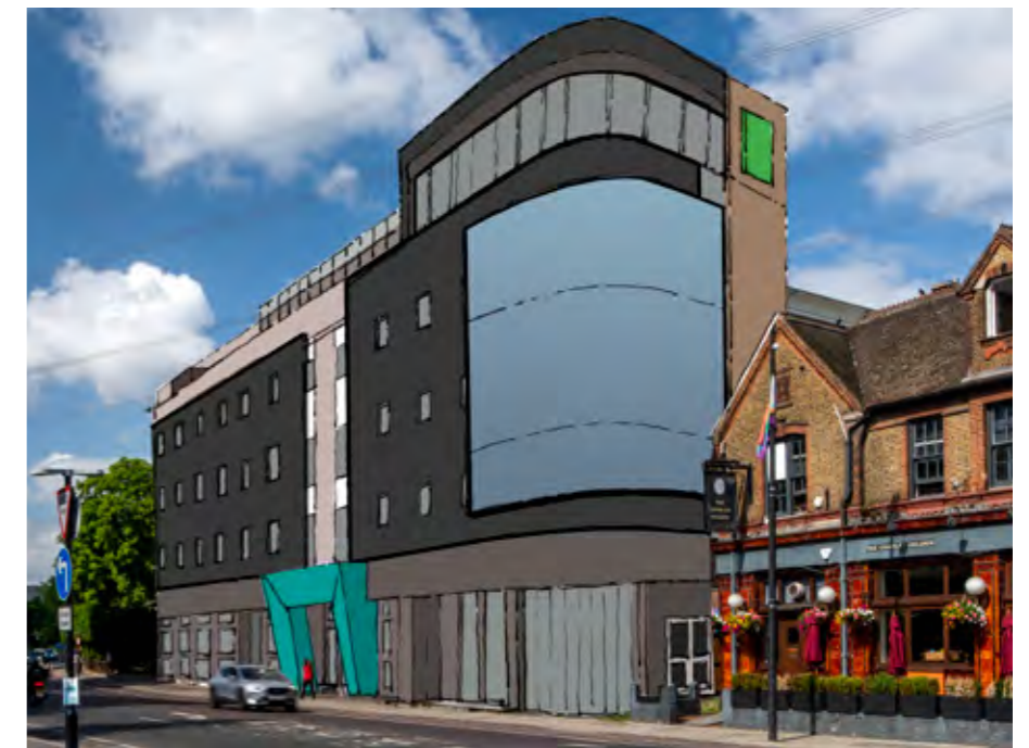
A projecting entrance surround has been implemented and a curved digital screen has been added to animate the corner of the proposed extension.
