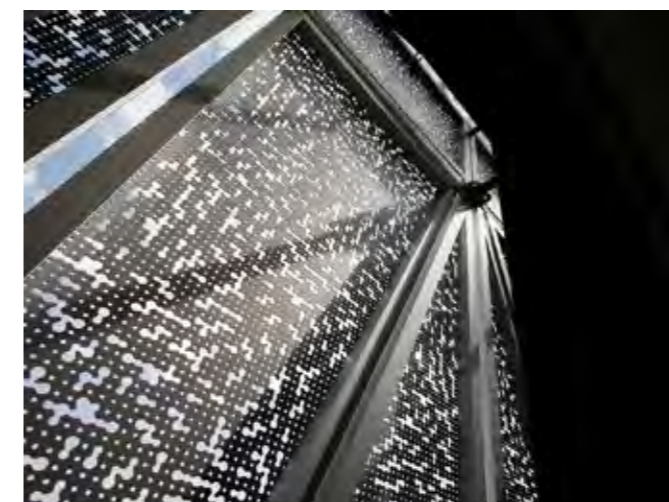
Perforated cladding over glazing
