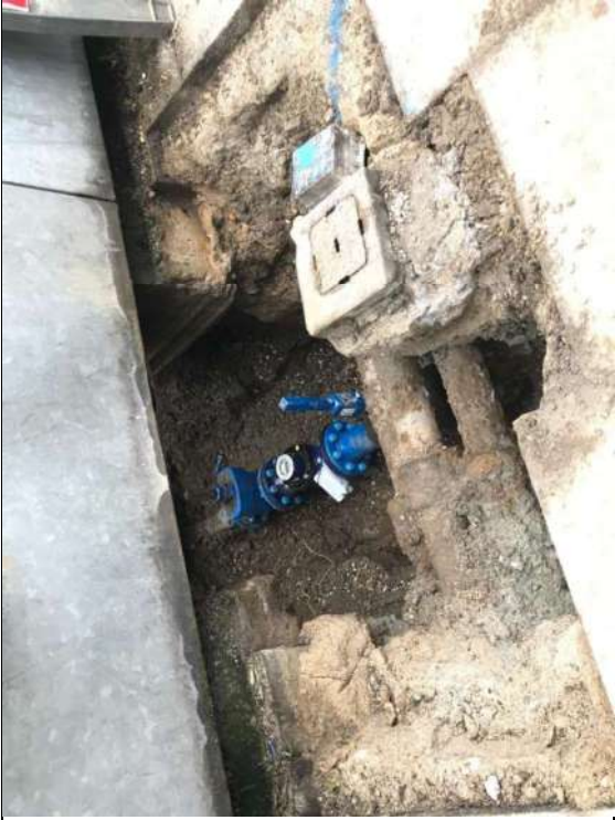
Plate 5: Groundworks (utilities) were taking place at the eastern corner of the PDA during our visit. Made ground was visible below the paving slabs.
