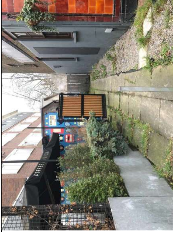
Plate 3: Facing down the northeastern edge of the PDA. Existing single storey café and substation are visible in this image.
