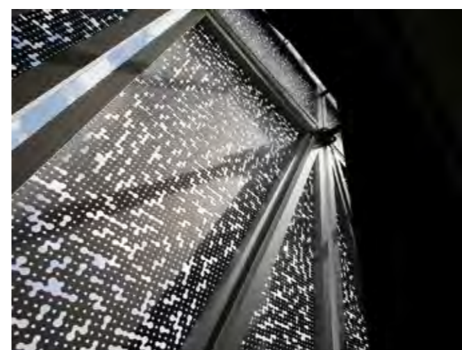
Perforated cladding over glazing
