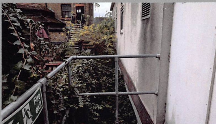
Shrubs to the north of the site
