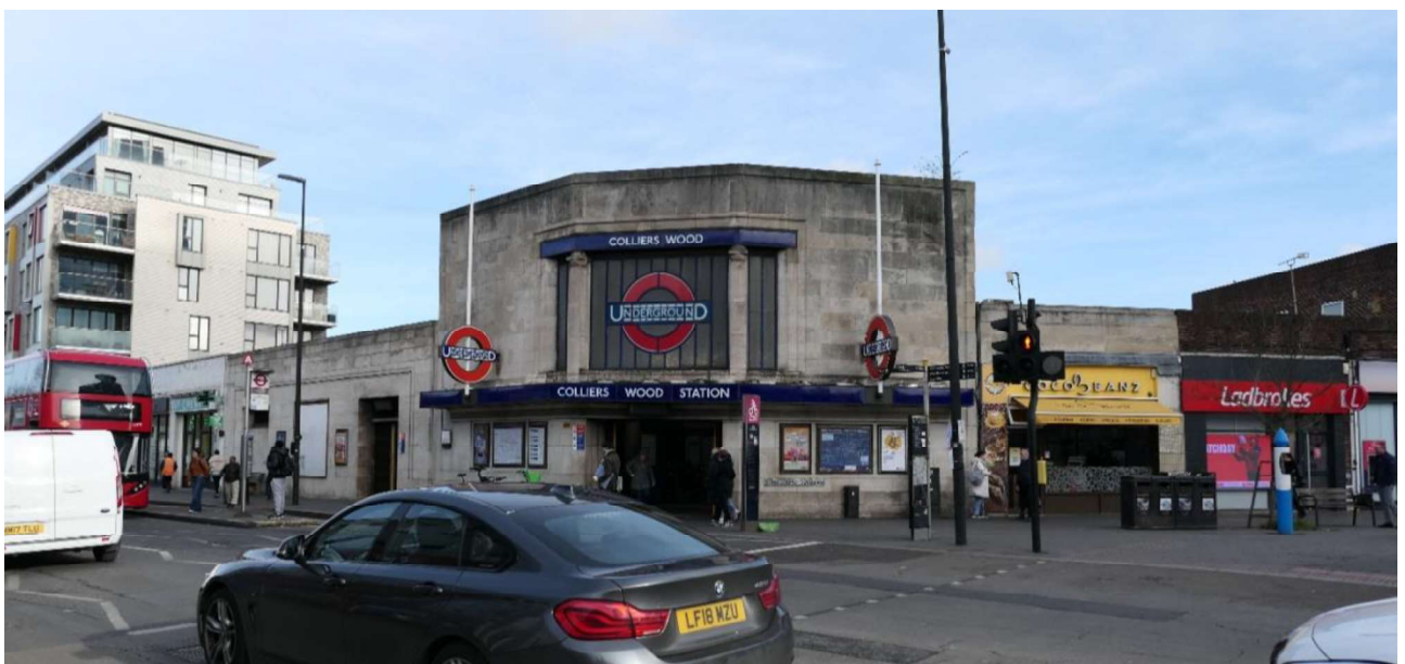
Photo 3: The grade II listed Underground Station.
