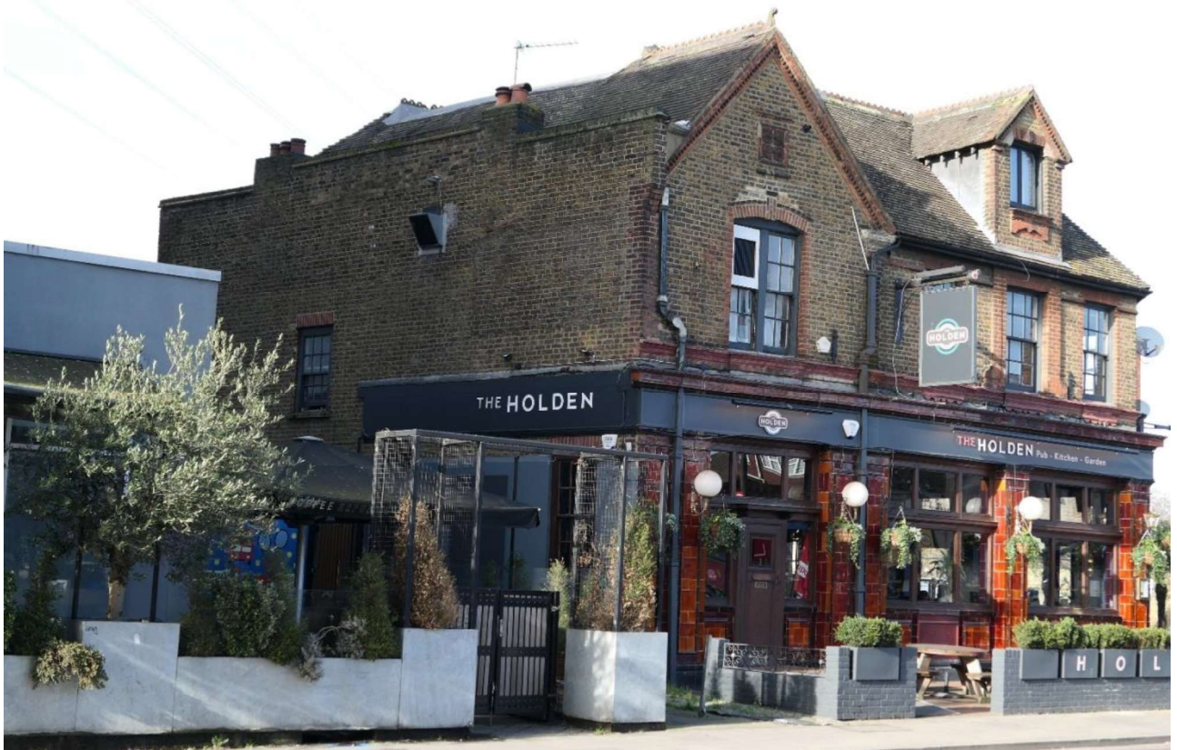
Photo 11: The southern elevation of the pub was originally blind (a window has been inserted later), and unlike the remainder of the building, it is plain.
