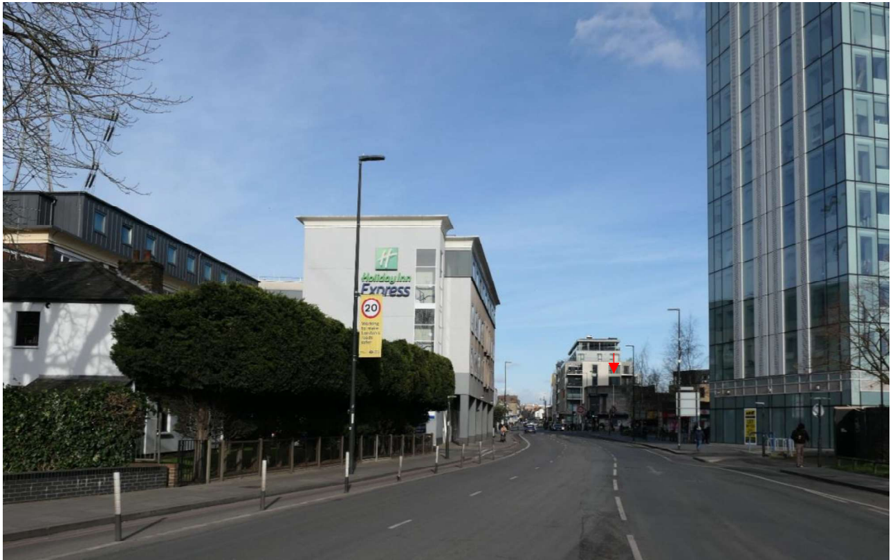
Photo 10: The Colliers Wood Underground Station (red arrow), seen in context with the present building on the application site and Britannia Point.
